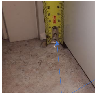
Approx. 4 mm difference across doors measured
