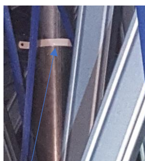
Flue through roof was correct
